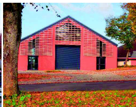
La halle multi-usages
